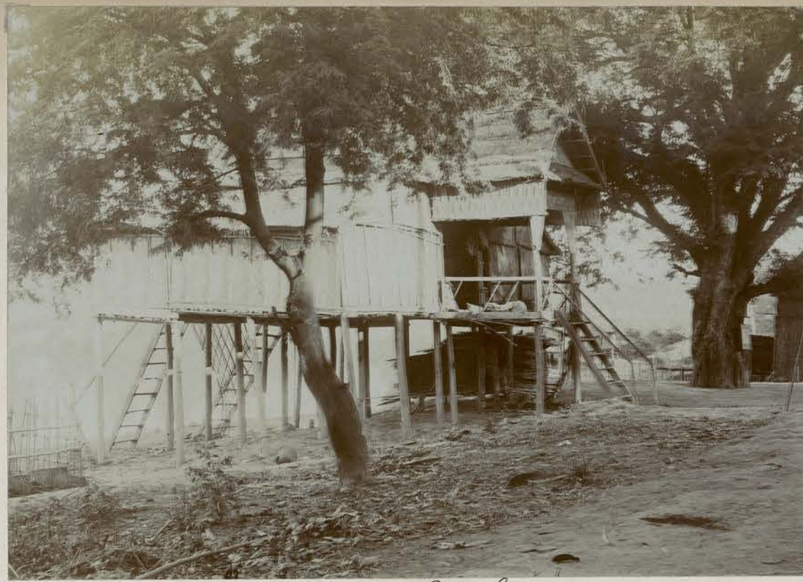
Resthouse; Pak Se.
