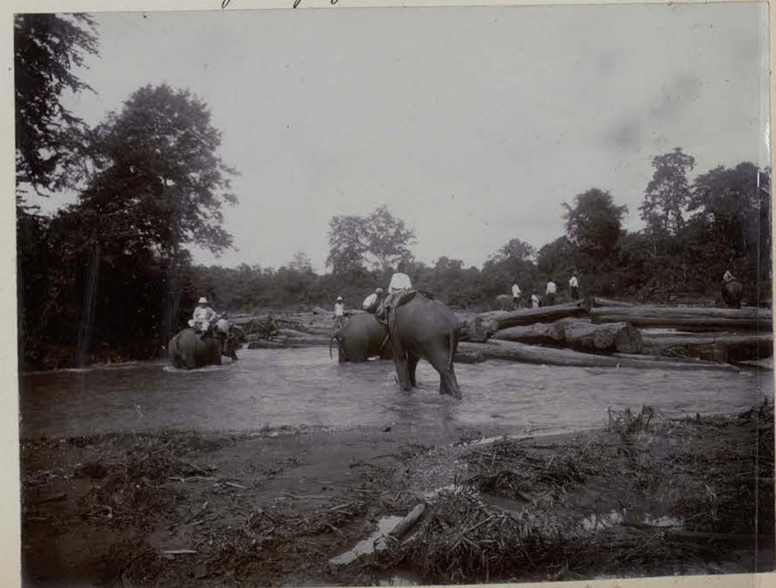
48 Splitting a pile 48
