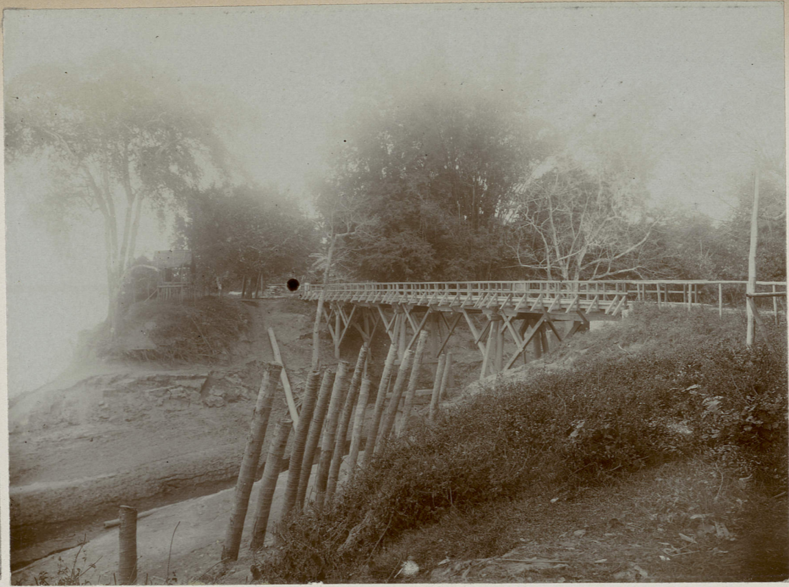
Bridge; Vieng Chan
